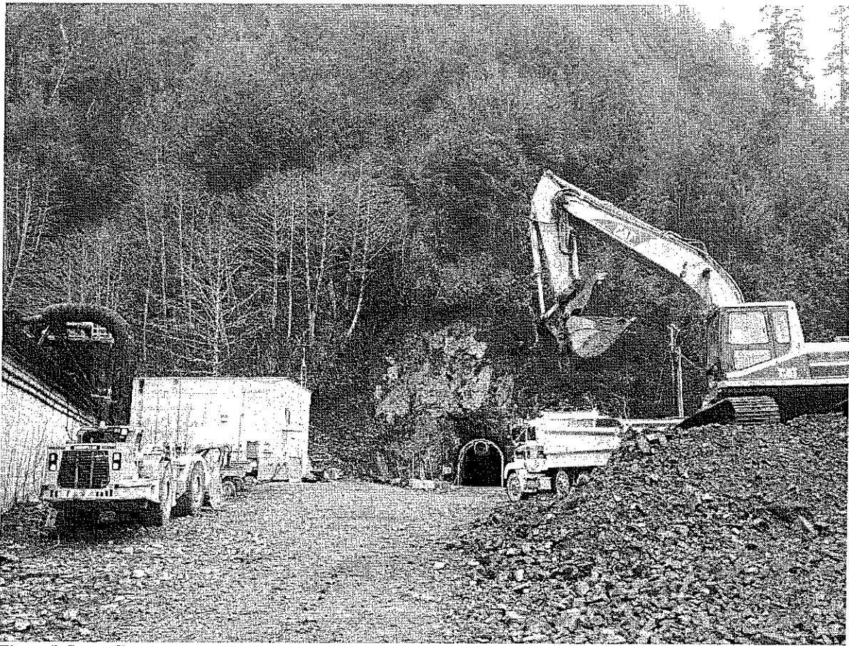
Figure 5. Surge Chamber Adit, the 470' adit tunnel was completed in late February.
