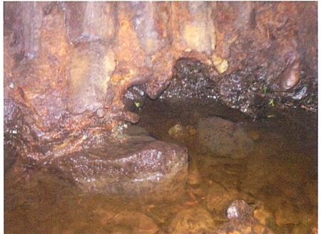
The middle third of the culvert is competent for the most part. These 5 photos were taken in about a 20-foot stretch of the pipe, starting about two-thirds of the distance upstream from the outlet, where the bottom of the pipe is gone.
