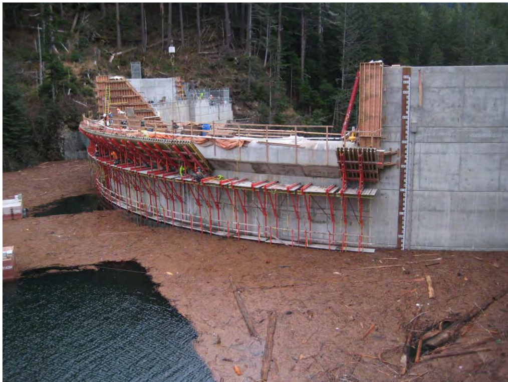
Figure 4: Upstream View of Dam Raise (WSEL 402)
