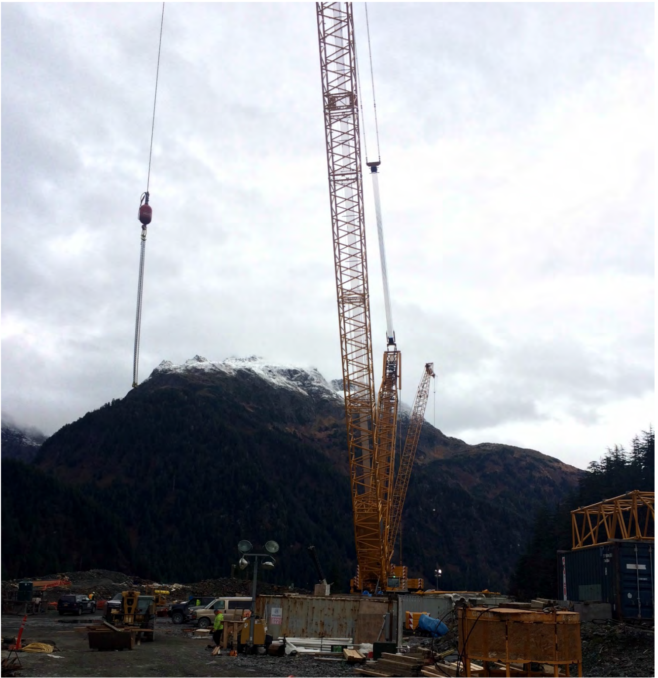
Figure 4. Dam Staging area, no change this month.
