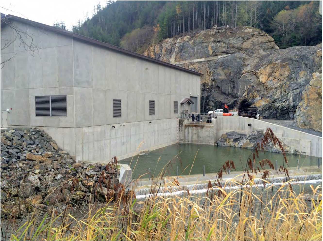
Figure 6. Powerhouse Site, no change this month.
