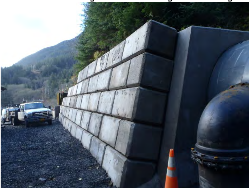
Figure 2: Ecoblock Wall at Penstock
