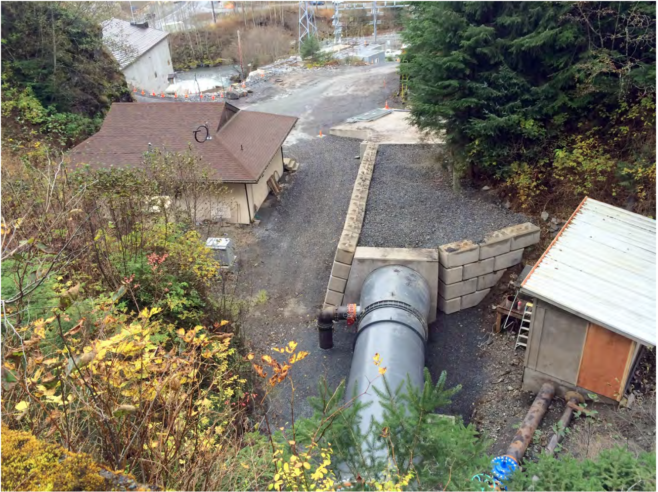
Figure 5. Lower Portal Area, Barnard completed Water Treatment Plant piping tests.
