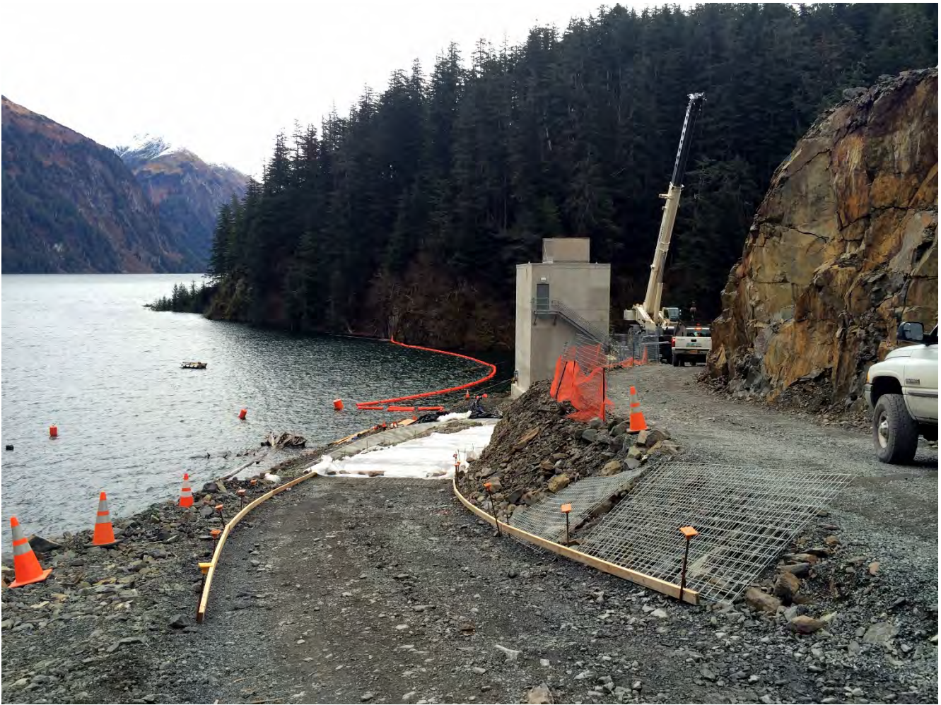
Figure 3. Gate House Location, Continued paving access road to the lake.
