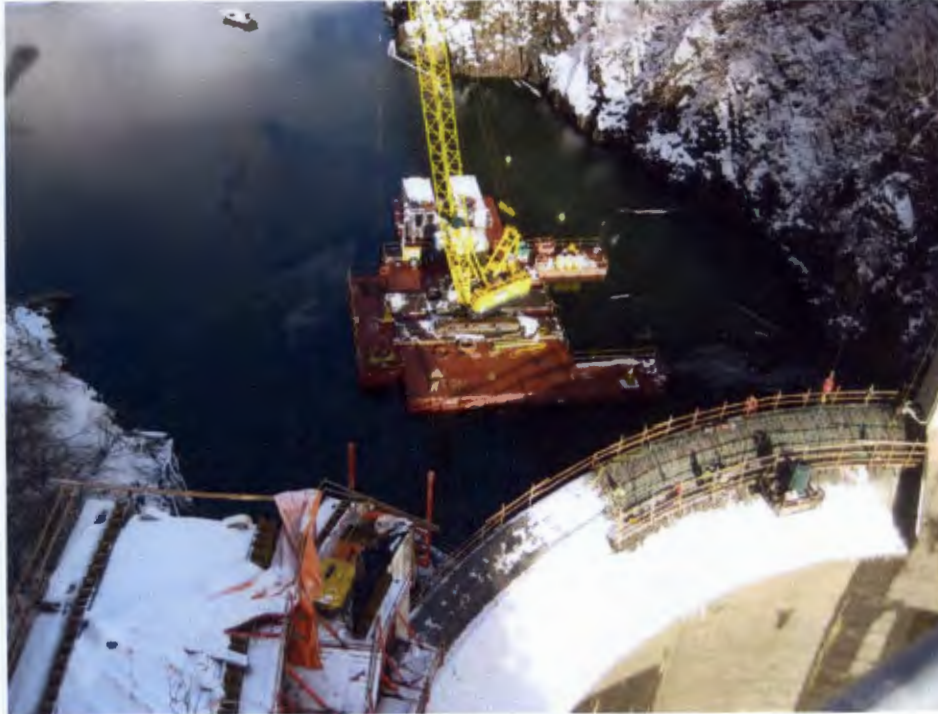
Figure 4: Spillway Keyway Construction
