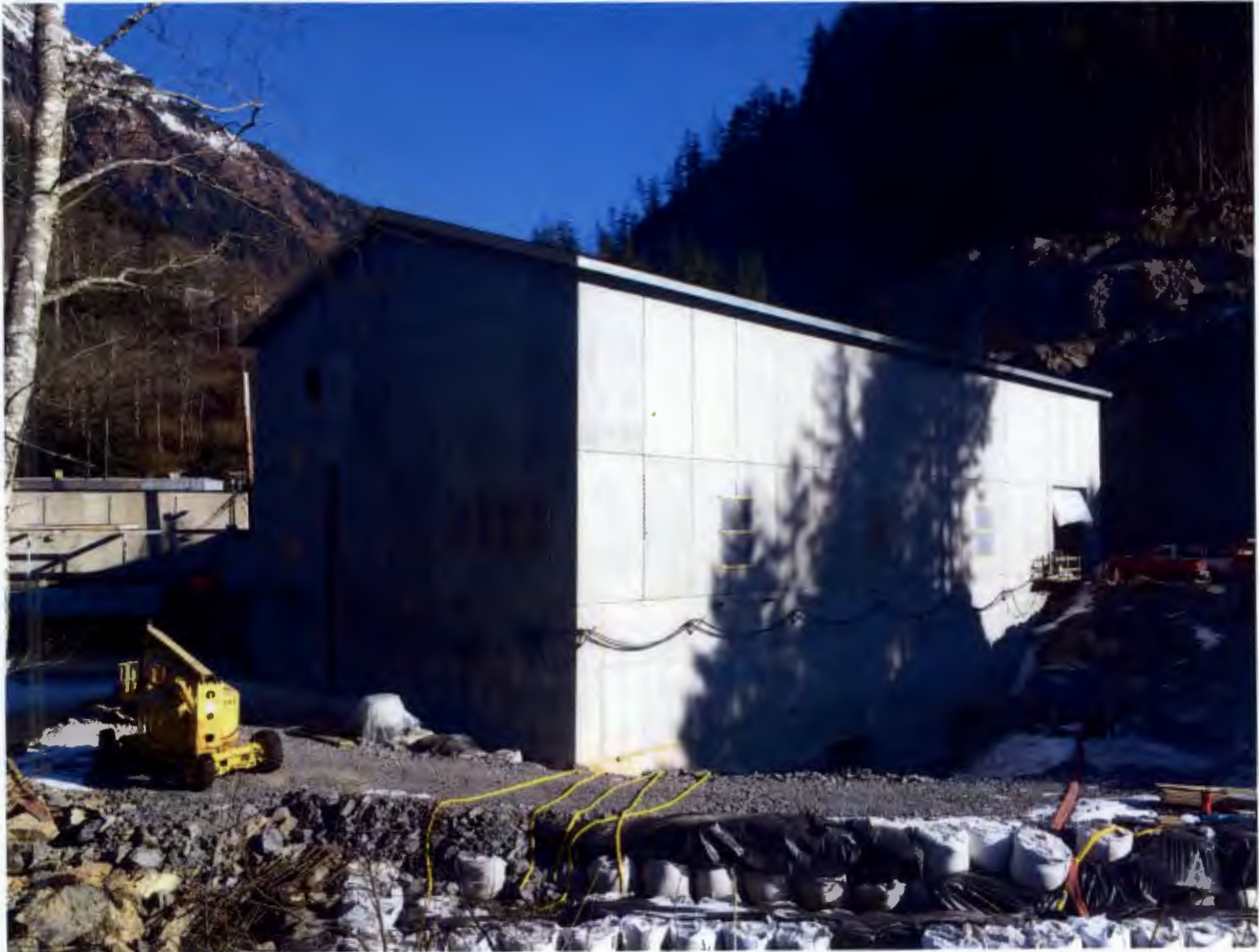
Figure 7. Powerhouse Site, The Powerhouse access road was completed.
