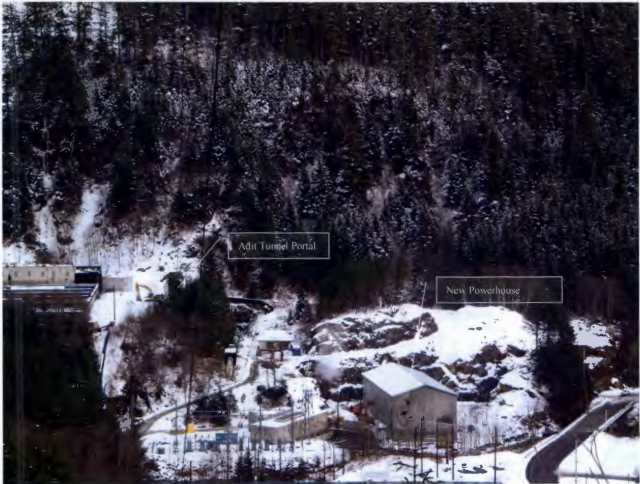
Figure 9. Lower Project Site, No change this month.
