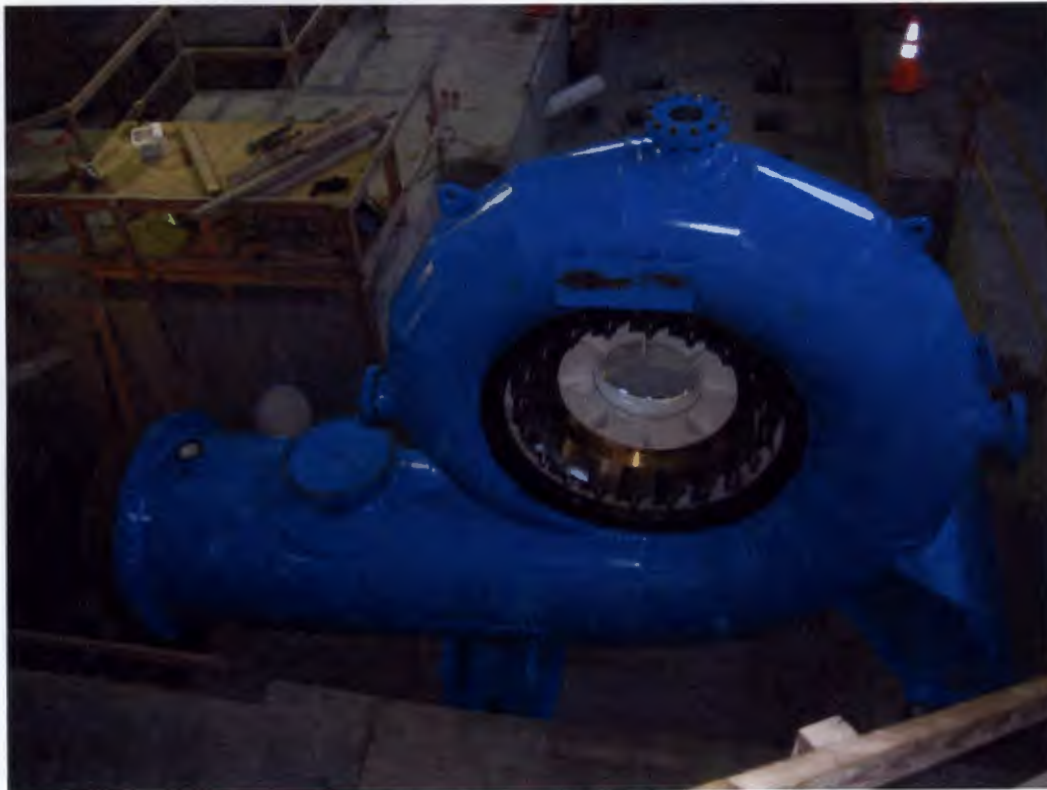
Figure 3: Unit 5 Spiral Case
