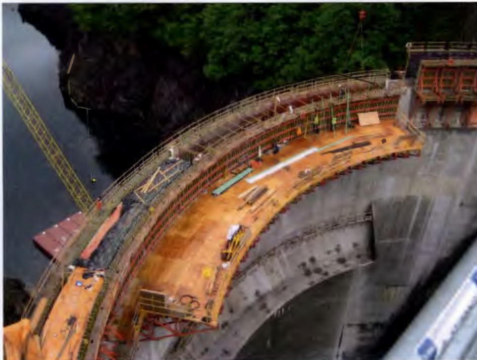
Figure 6: Dam Raise and Spillway Shoring Deck
