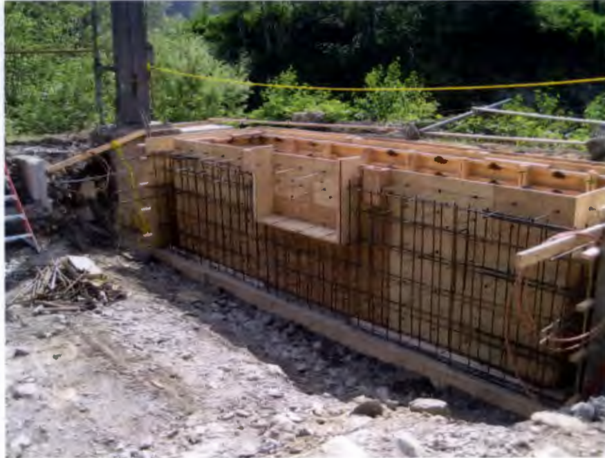
Figure 5: T1 Transformer Foundation
