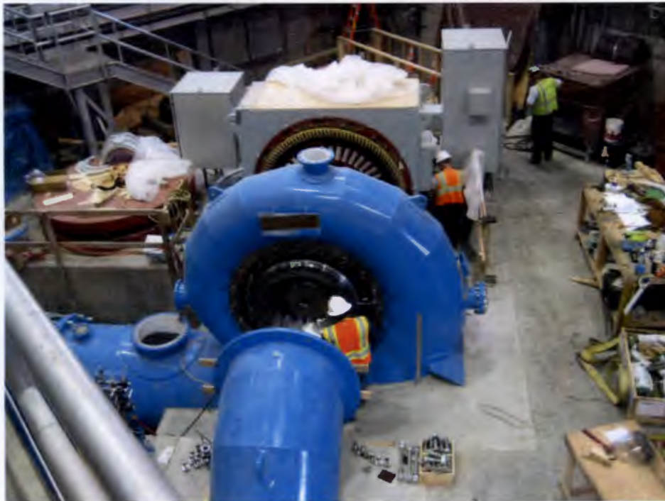
Figure 2: Unit 3 Rotor Alignment
