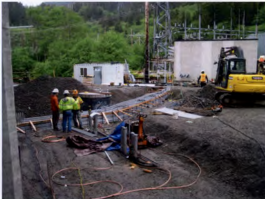
Figure 4: Duct Bank and SST Foundation
