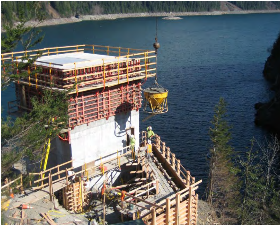
Figure 2: Gatehouse Retaining Wall Placement
