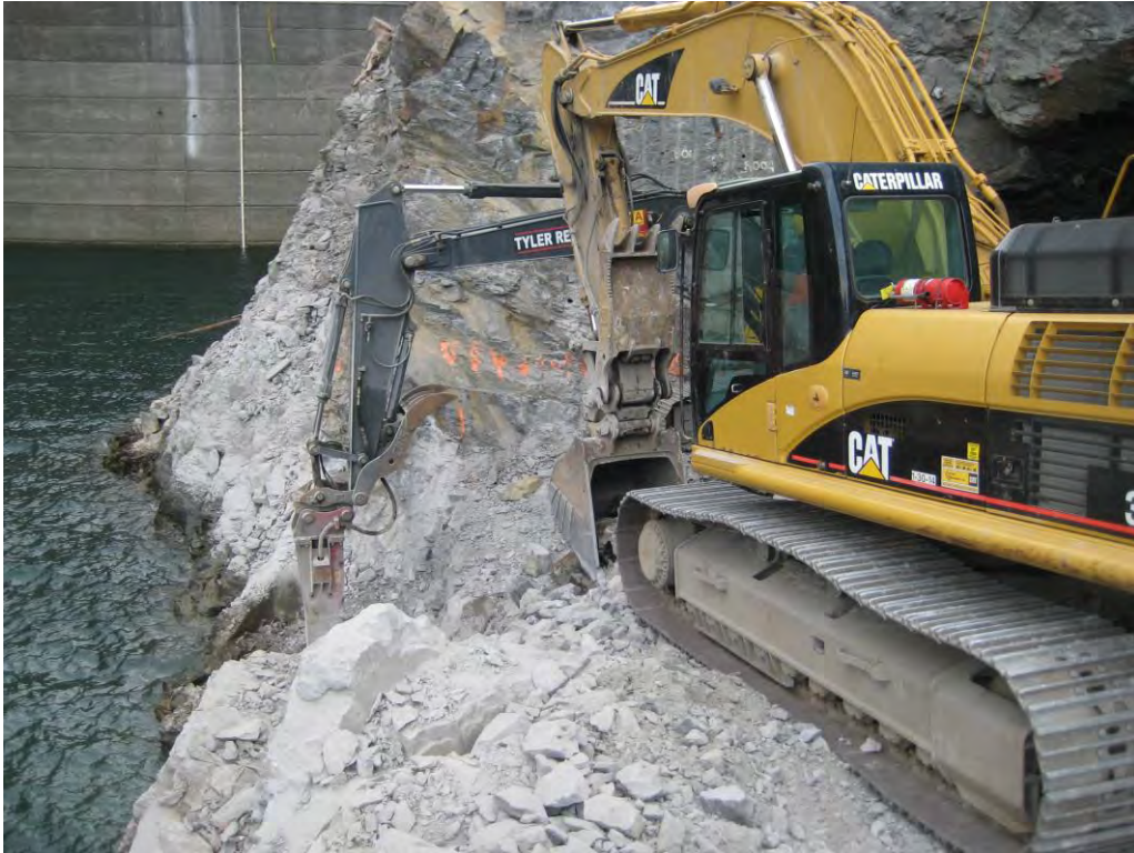
Figure 3: Intake Structure Excavation
