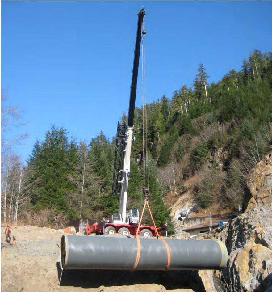
Figure 6: Staging Penstock Pipe
