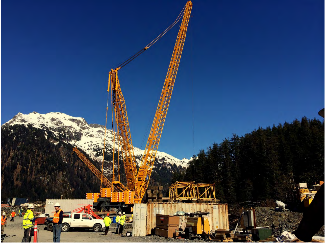
Figure 5. Dam Staging area, a new smaller 150 ton Liebherr crane was set up to assist with the dam raise.
