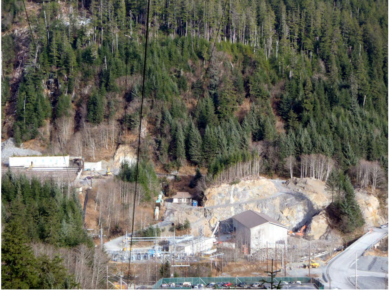
Figure 8. Lower Project Site, No change this month.
