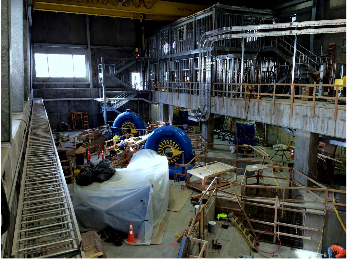
Figure 9. Powerhouse Interior, Schmolk began the powerhouse mechanical rough-in. Completed final alignment of BLU unit 5 turbine spiral case and grouted in place. Placed BLU unit 5 turbine draft tube. Completed final alignment of BLU-5 sole plates and epoxy grouted the anchor bolts. NAES continued with installation of conduit and cable tray in powerhouse and installed conduit for lighting and plant services. ASRC continued framing and building out the control room.
