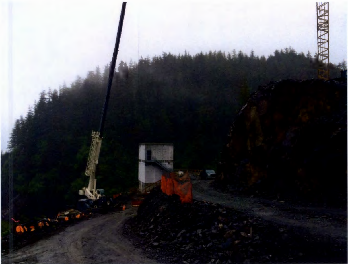
Figure 4. Gate House Location, Barnard, NAES, and Schmolk continue the inside build out of the gate house.
