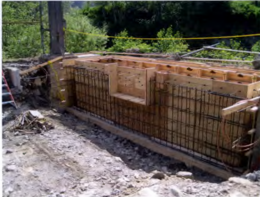
Figure 5: T1 Transformer Foundation
