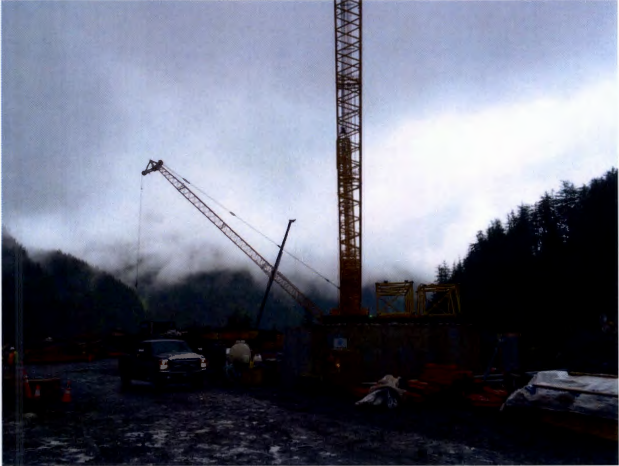
Figure 5. Dam Staging area, no change this month.
