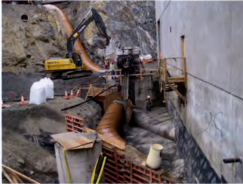
Figure 3: CDF Backfill on Lower Penstock
