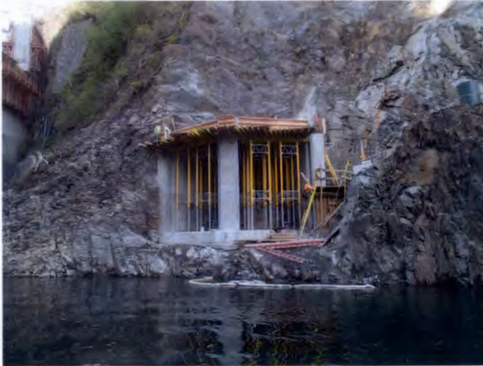
Figure 7: Intake Structure
