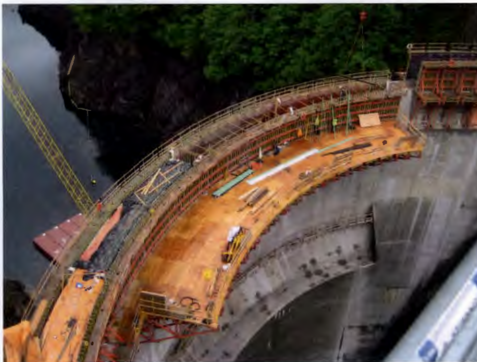
Figure 6: Dam Raise and Spillway Shoring Deck
