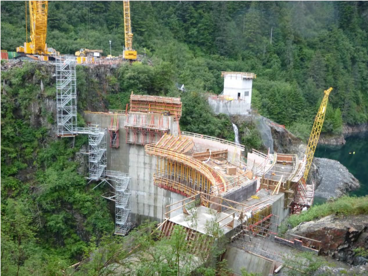
Figure 3. Intake Portal and Right Abutment, The new intake structure is 90% submerged. Crux completed all but 6 curtain grout holes on the right abutment.
