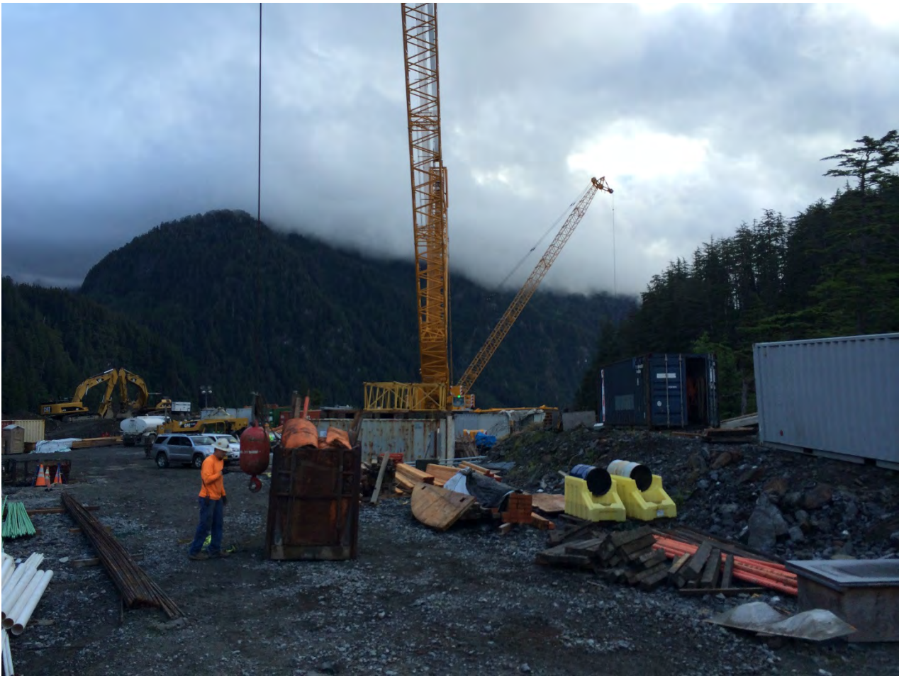
Figure 5. Dam Staging area, no change this month.
