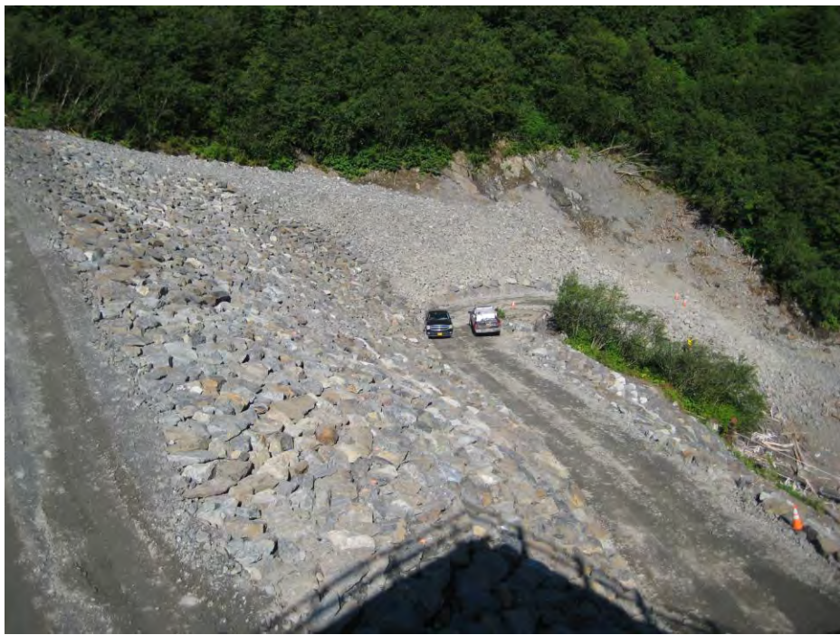
Figure 5: Completed Reservoir Access Road
