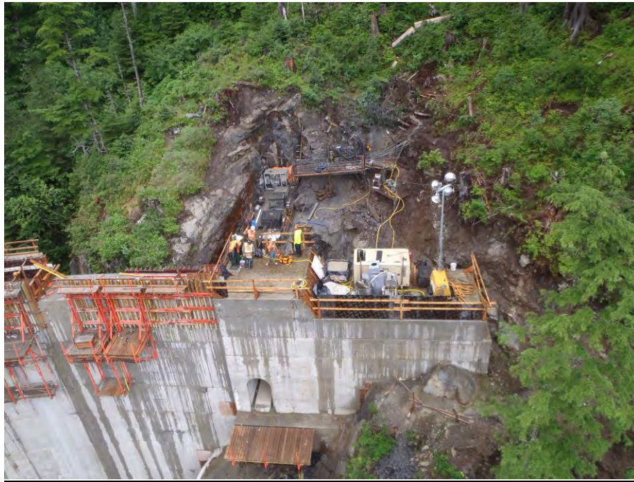
Figure 2: Left Abutment Curtain Grouting
