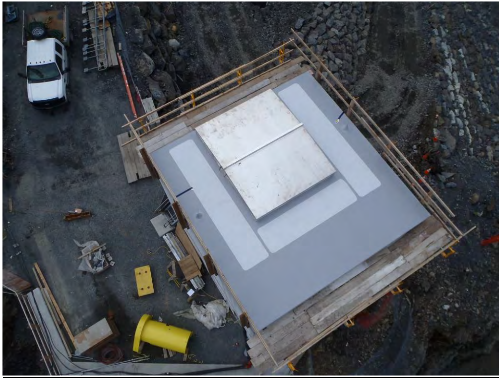
Figure 4: Gate House Roof and Hatch
