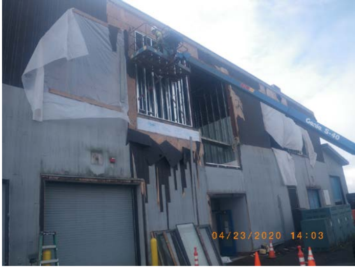
Exterior siding demo
