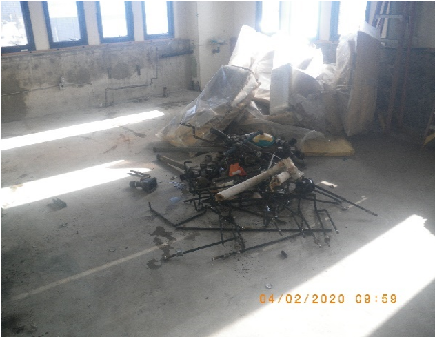
Copper pipe demo in the lab
