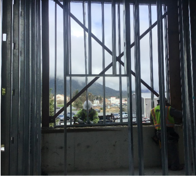
New interior framing
