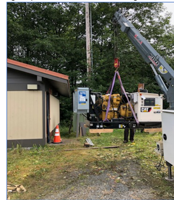
Hoisting the New Halibut Point Generator
