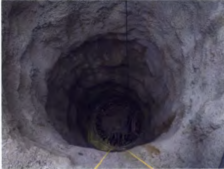
Figure 3: Gate Shaft Liner Formwork
