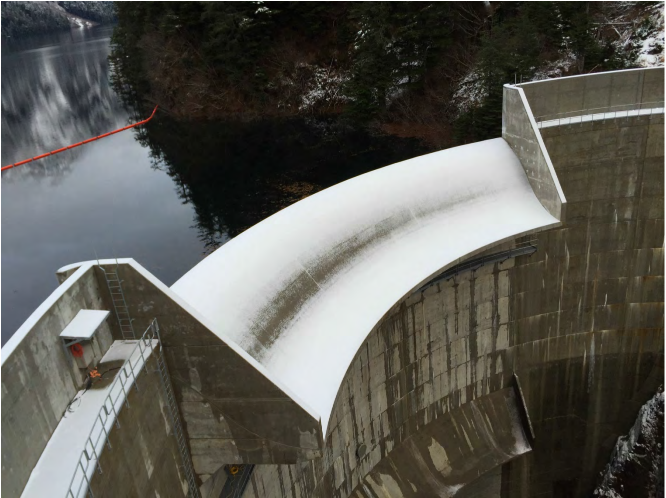
Figure 1. Dam and Left Abutment Area, Barnard crews removed all concrete forms.
