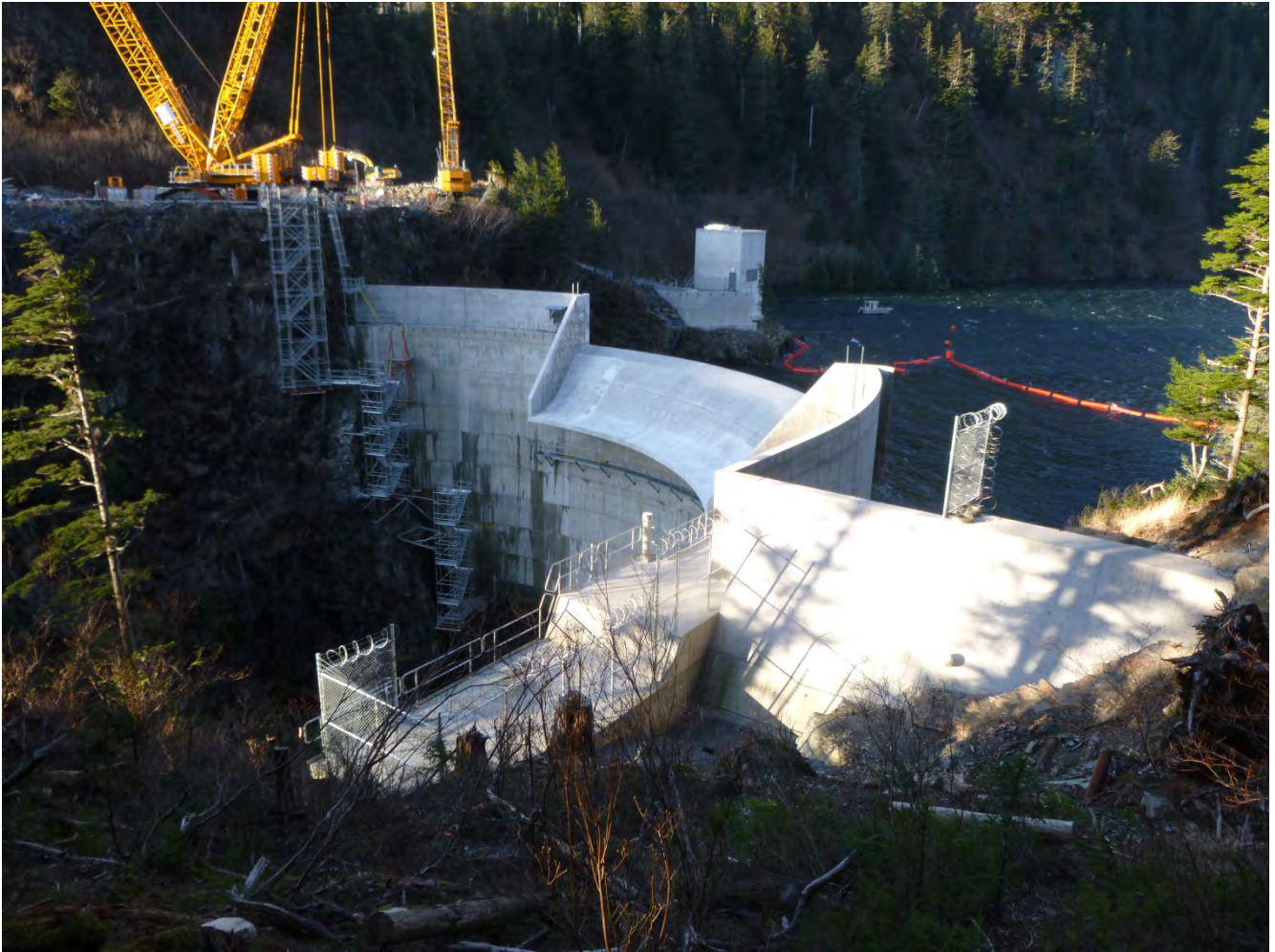
Figure 2. Intake Portal and Right Abutment, Spillway sack and patch work completed.
