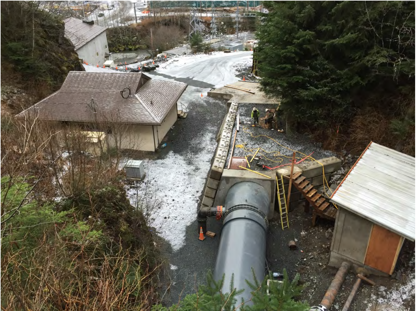
Figure 5. Lower Portal Area, Final fill is being placed on the penstock.
