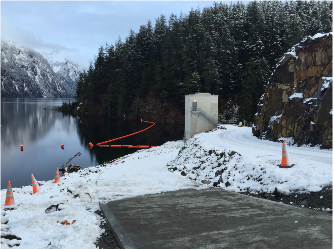
Figure 3. Gate House Location, Reservoir access road paving completed.
