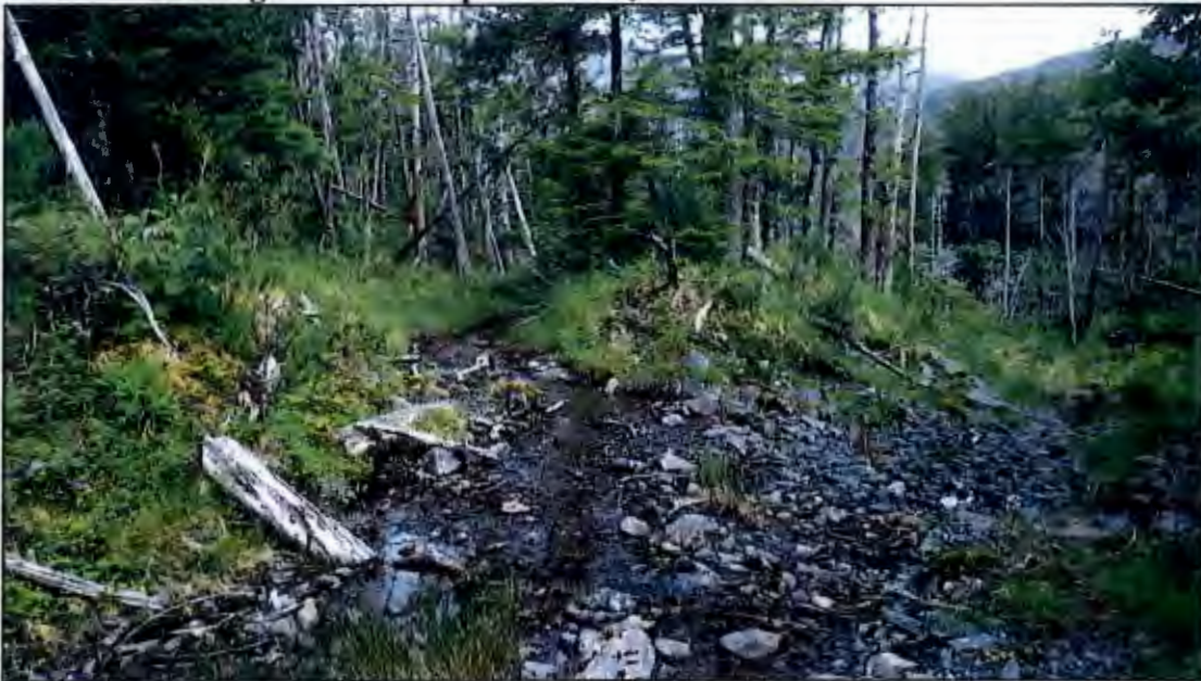
Photo H. Looking downhill on spur road #1, 50' above Photo G.
