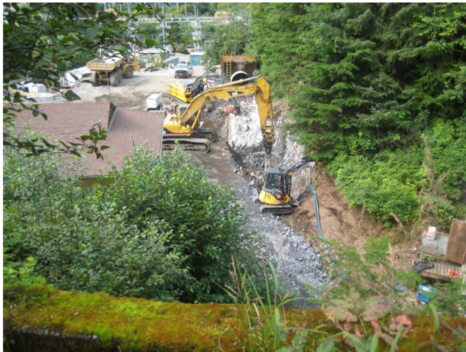
Figure 5: Penstock Excavation
