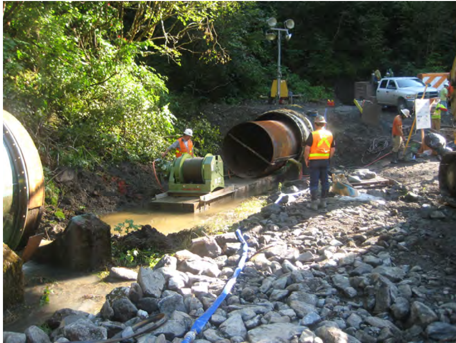
Figure 4: South Portal Liner Installation
