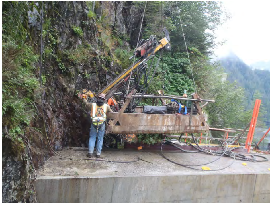
Figure 3: Right Abutment Curtain Grouting
