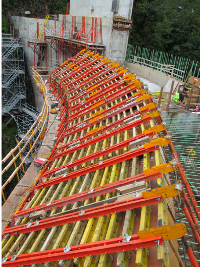
Figure 1: Spillway Formwork
