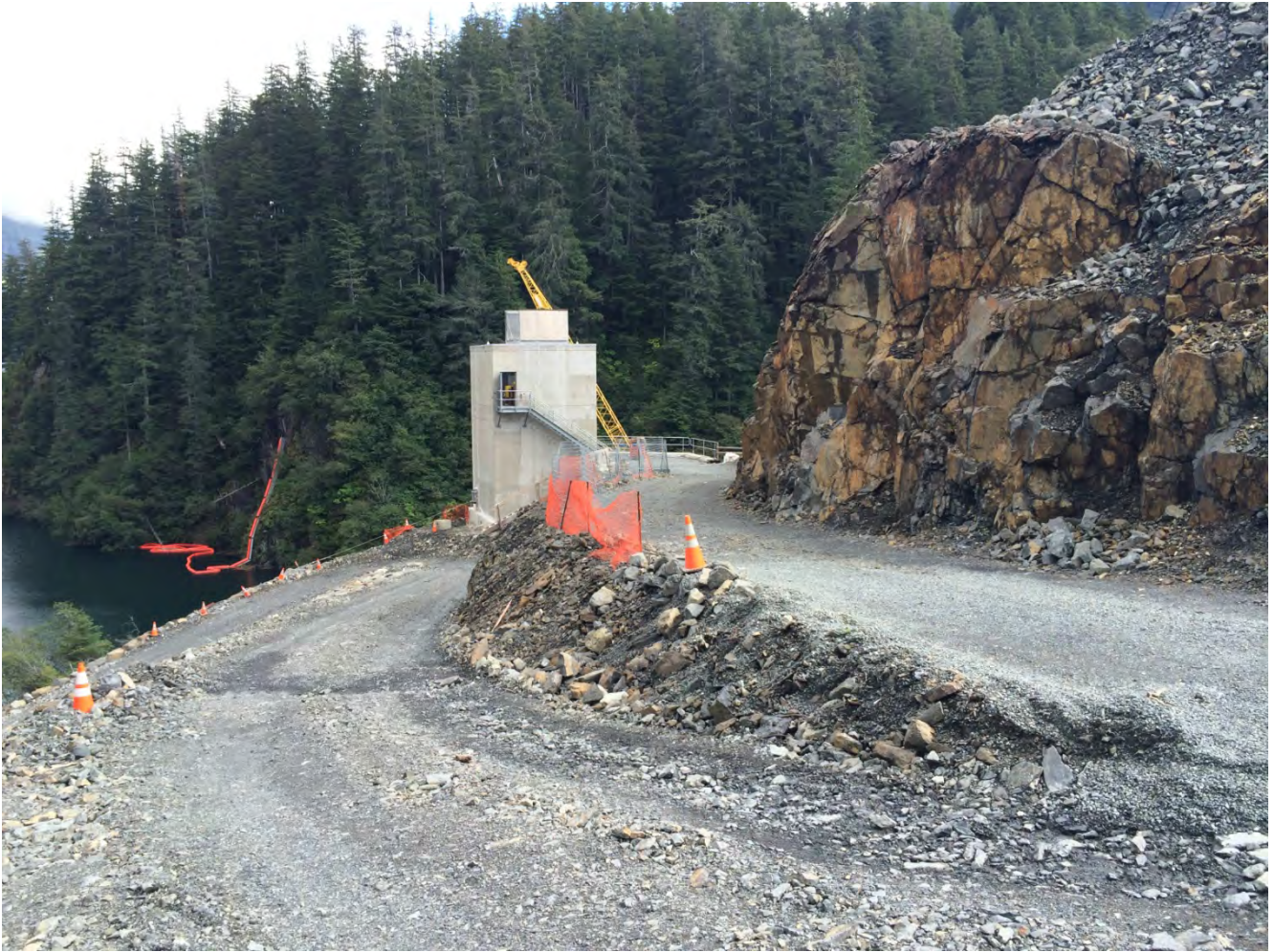
Figure 3. Gate House Location, Completed dry testing of the fixed wheel gate.
