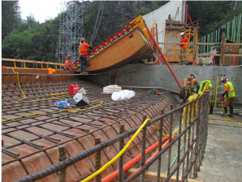
Figure 2: Rebar and Formwork for M4/410
