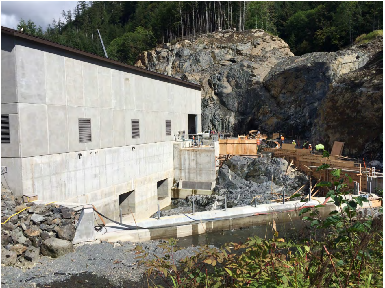
Figure 7. Powerhouse Site, AMCL continued work on the raw water intake and after bay.
