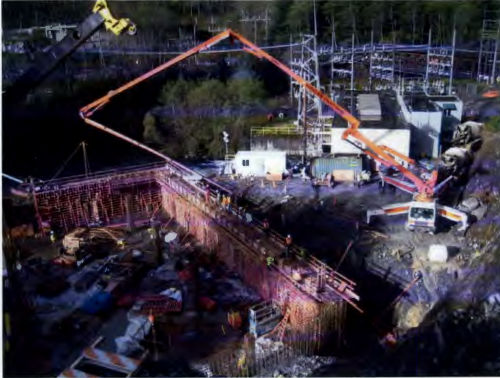
Figure 3: Powerhouse Walls Placement
