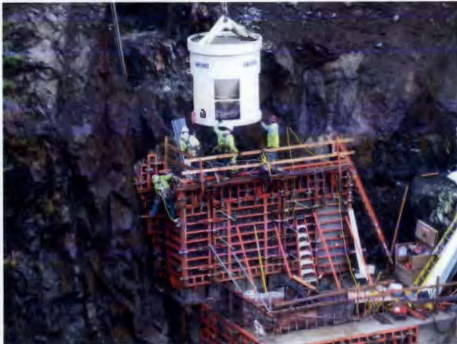
Figure 4: Cutoff Wall Concrete Placement
