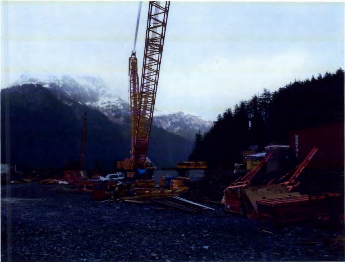
Figure 5. Dam Staging area, No change this month.
