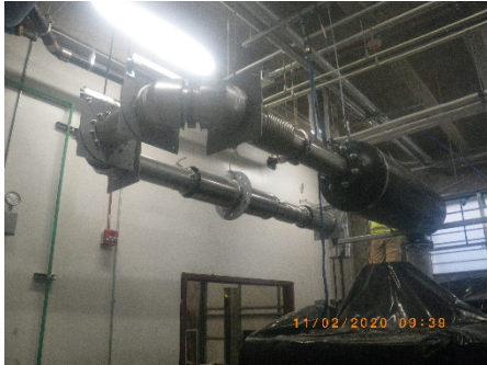
Stand-by generator exhaust pipe installation
