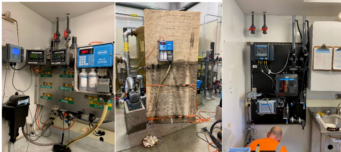
Photos: Antiquated analyzers, temporary chlorine analyzer, skid-mounted analyzers being installed
