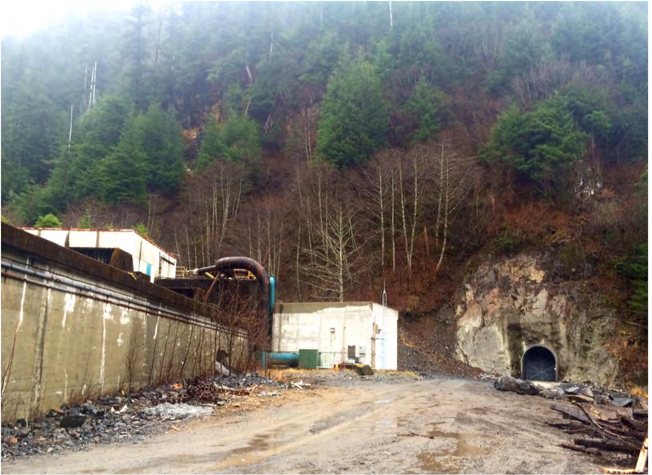
Figure 8. Surge Chamber Adit, Complete.
