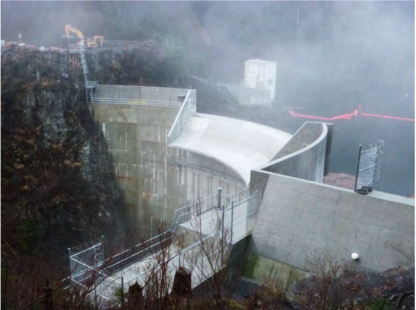
Figure 2. Intake Portal and Right Abutment, Complete.
