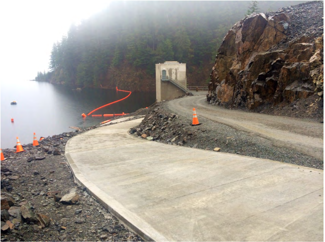
Figure 3. Gate House Location, Complete.
