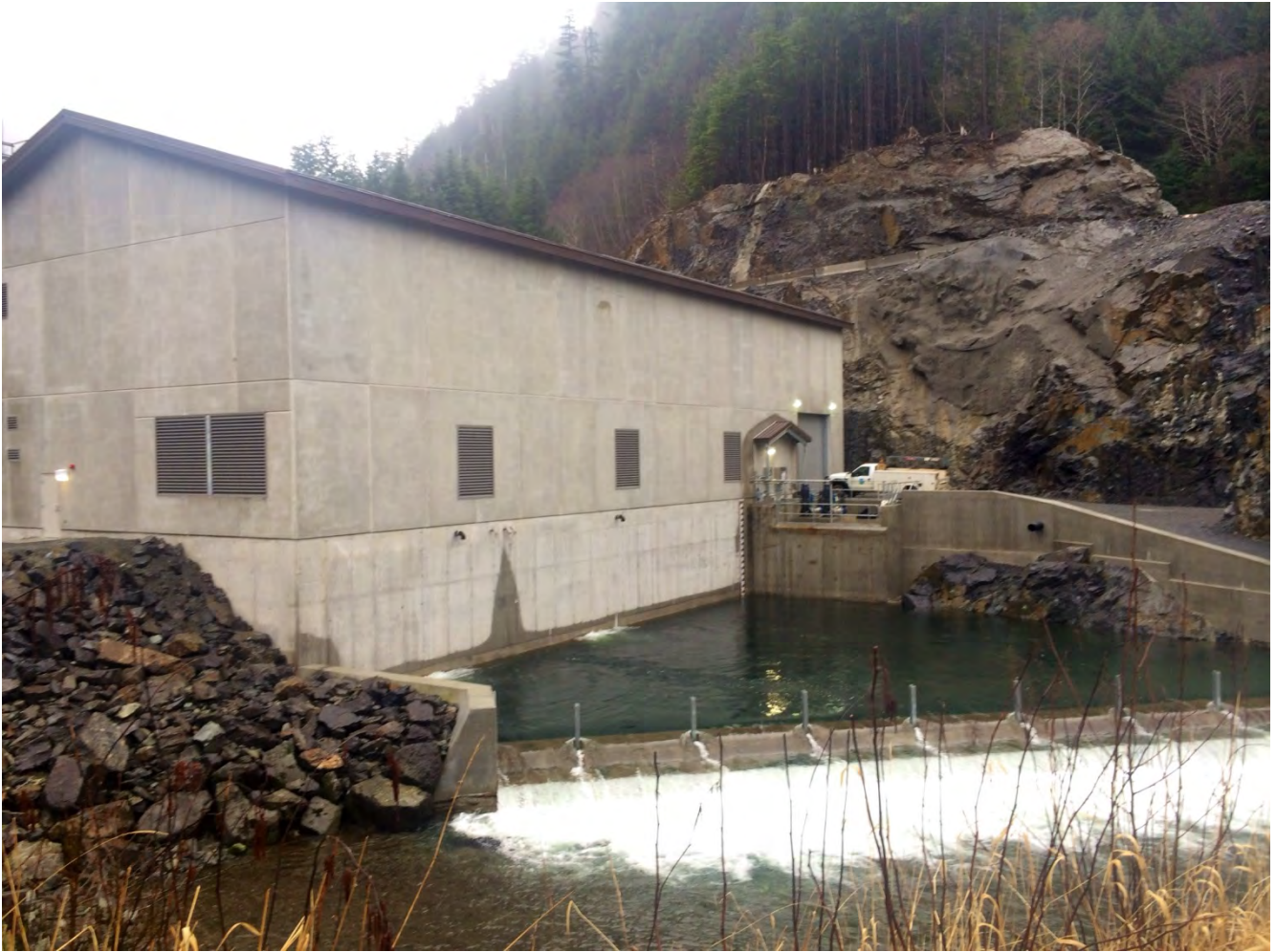
Figure 6. Powerhouse Site, Complete.
