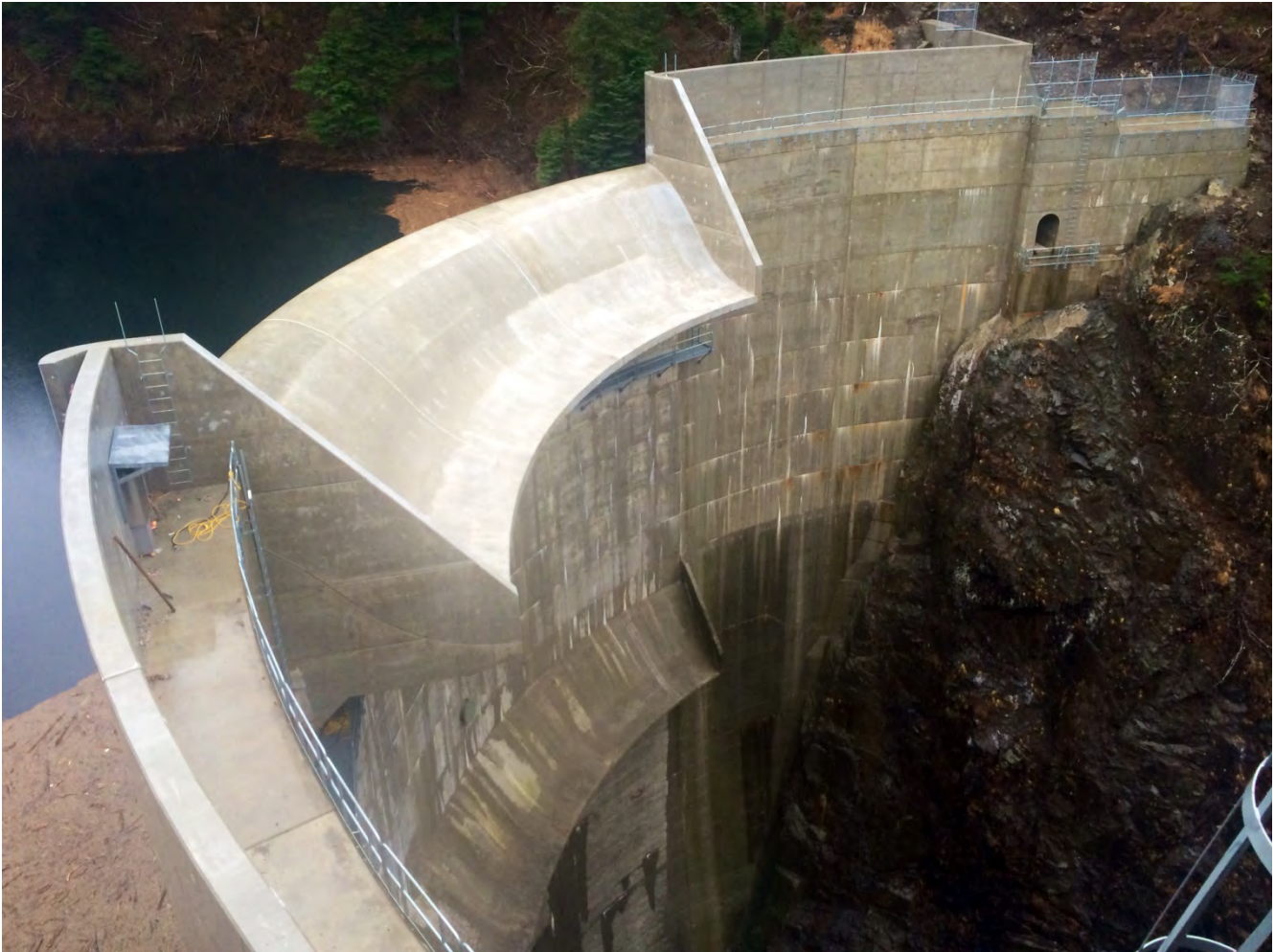
Figure 1. Dam and Left Abutment Area, Complete.
