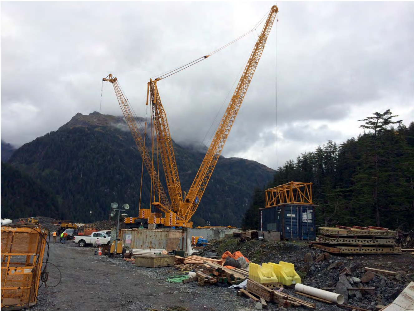
Figure 4. Dam Staging area, no change this month.
