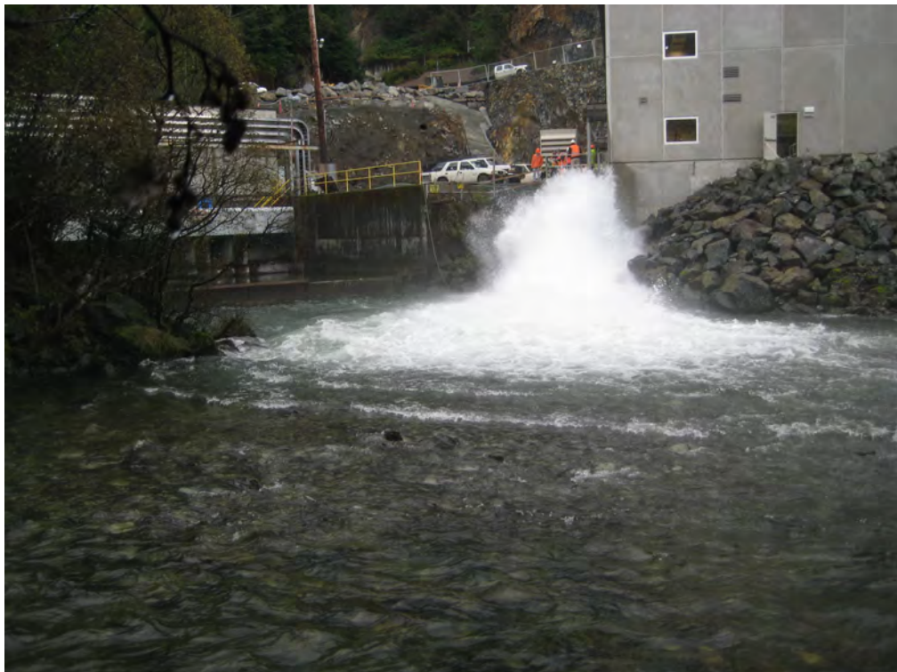
Figure 4: Penstock Drain Testing
