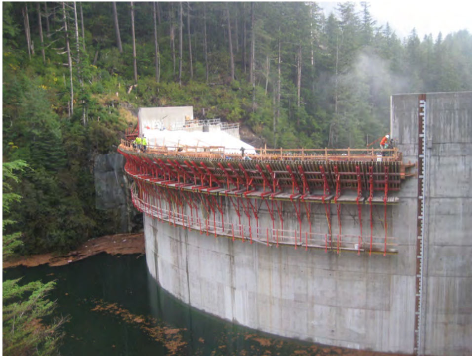
Figure 2: M4 Spillway Finish
