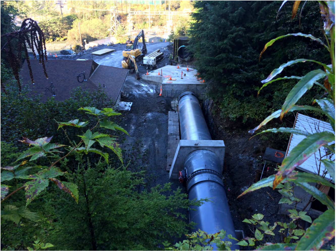
Figure 5. Lower Portal Area, Penstock anchor block 5 was completed.
