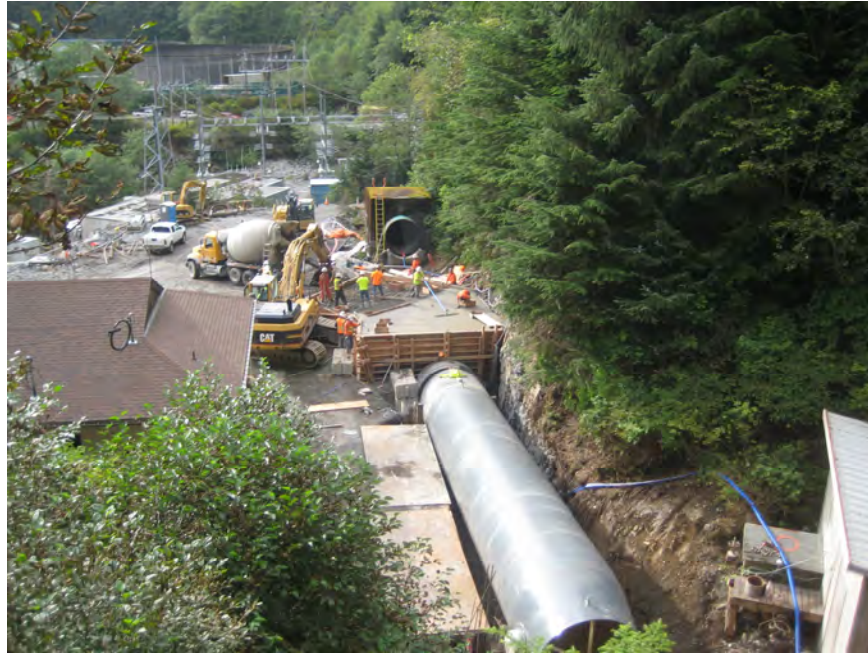
Figure 3: Lower Portal and Anchor Block #5
