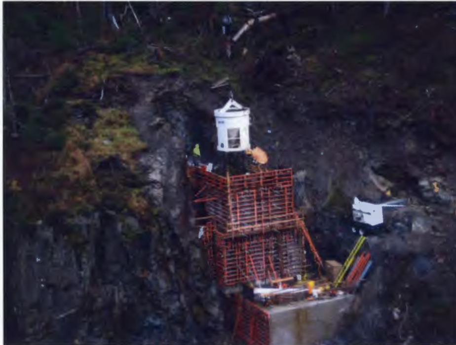
Figure 1: Cutoff Wall Concrete Placement
