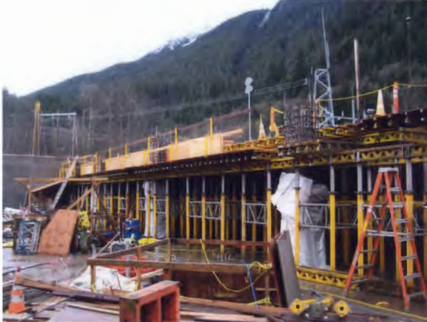
Figure 5: PH Mezzanine Deck Formwork
