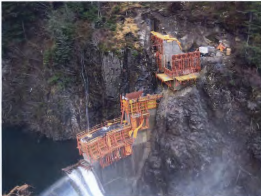
Figure 2: Dam Raise and Left Abutment
