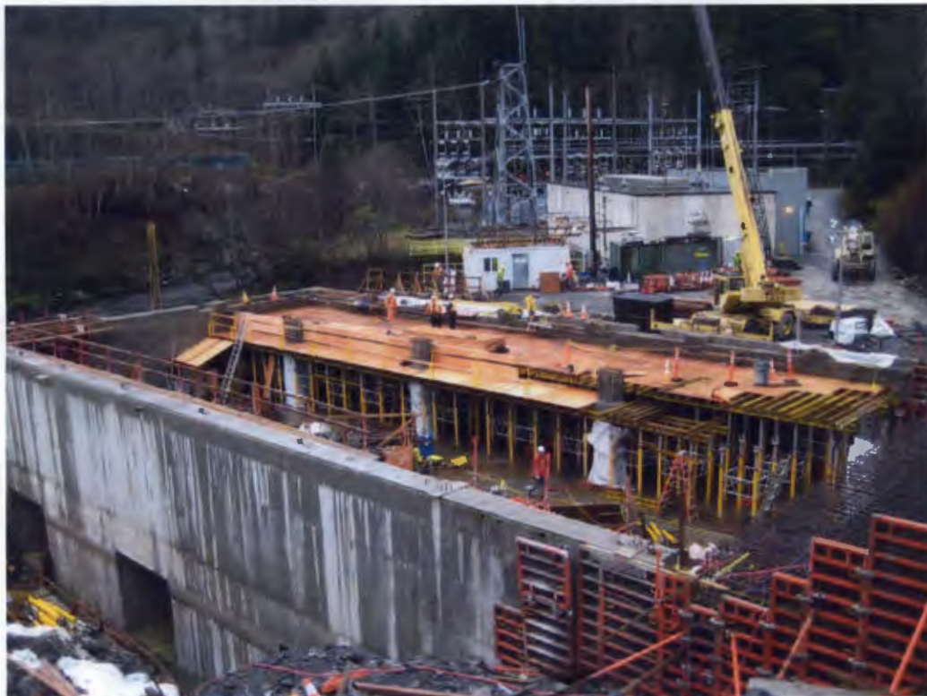
Figure 4: PH Mezzanine Deck and Access Bay
