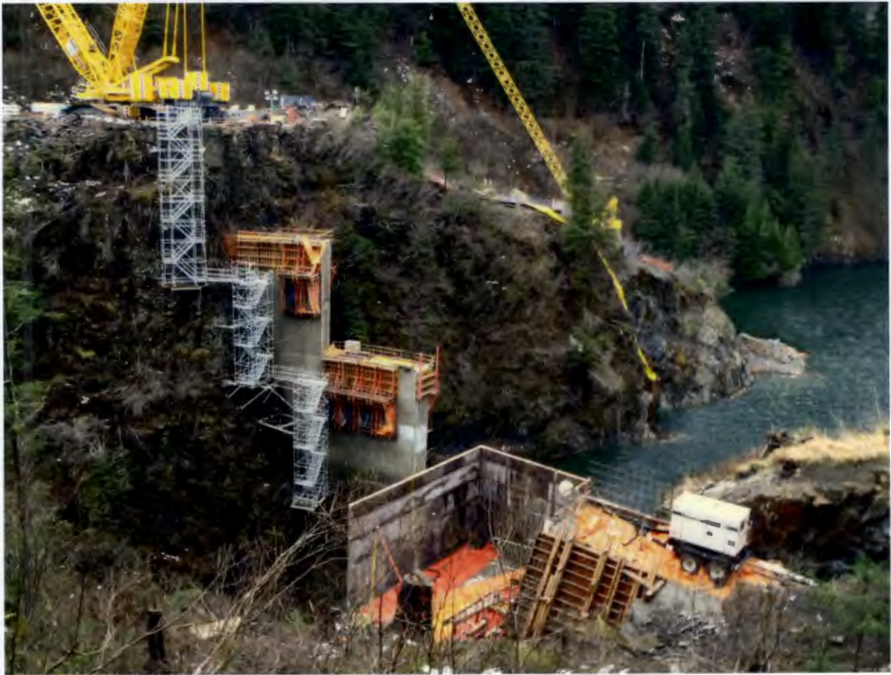
Figure 3. Intake Portal and Right Abutment, no change this month.
