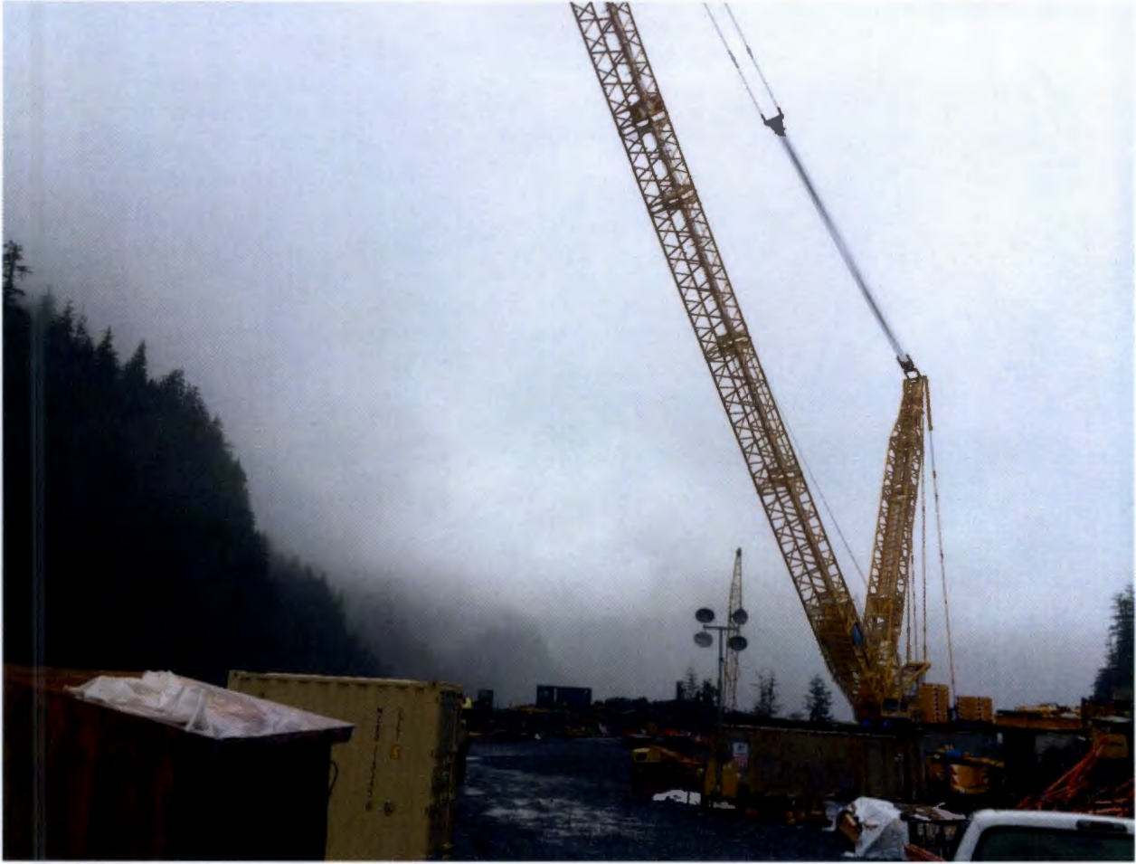
Figure 5. Dam Staging area, No change this month.
