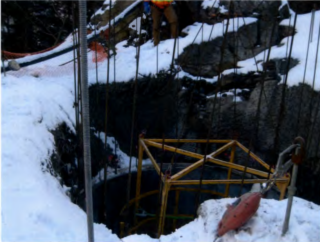
Figure 5: Gate Shaft Concrete Liner
