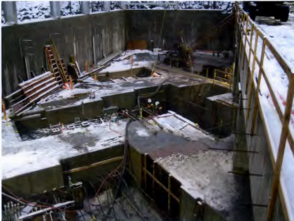
Figure 4: Powerhouse Turbine Pits
