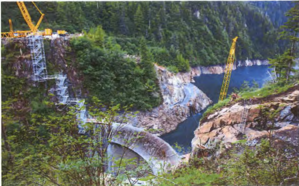
Figure 1 - Blue Lake Dam Construction
